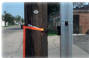
3 - Secure lift to pole
